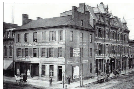
Above: Intersection of Second (right) and Paint (left), circa 1880. The Ross County Bank is the building at the right. None of the buildings pictured remain.
